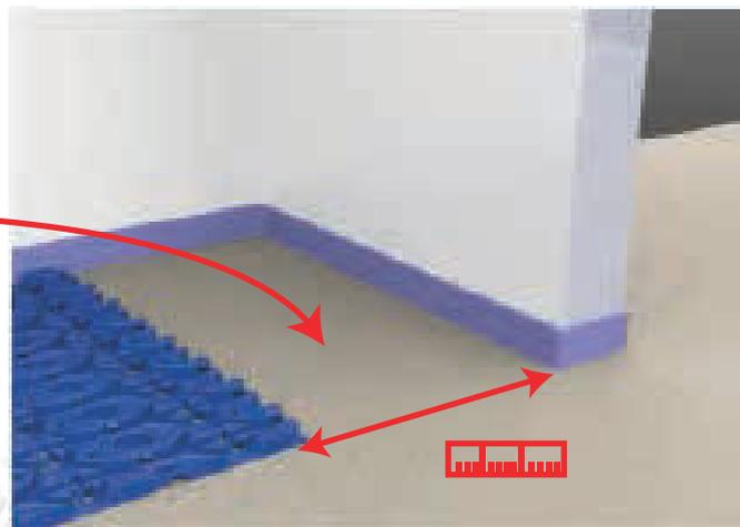
When you reach the edge of the room, measure the remaining distance and score the back of the panel using one of the pre-grooved cutting lines.
