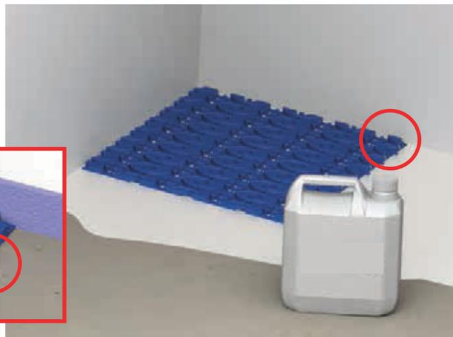
Mechanically fix the panels to the floor
