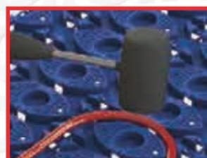
Ideally use a rubber mallet to fully engage the pipe work in place
